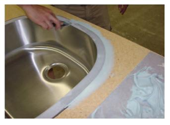
Mix up Bondo or similar body filler product. Smear Bondo into the gap around the sink. Fill the gap between sink rim and substrate completely. Leave to harden for about 10 minutes.
