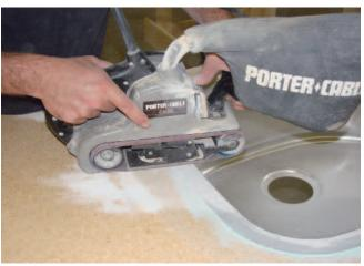
Once hard, use a belt sander with a coarse grit sandpaper to sand the rim of the sink and the Bondo. Make sure to keep the sander level so as not to sand the substrate or sink rim unevenly. Marking pencil lines on the rim and substrate is a useful guide to show high spots. Sand until lines have been removed.
