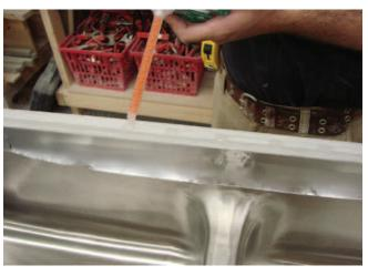
Prepare solid surface seaming adhesive. Remember to purge tube to ensure adhesive is mixing with catalyst. Apply a continuous bead about 1/8" back from the inner front edge of the sink. Bead should be between 1/4" and 3/8" wide. Then place small dots on outside of bead every 2" to 3". Use a color that is appropriate for the color of solid surface being used.
