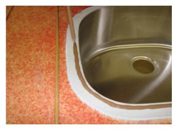
Prepare Karran Seaming Adhesive. Remember to purge tube to ensure adhesive is mixing with catalyst. Apply a continuous bead about 1/8" back from the inner front edge of the sink.
