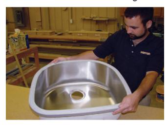
After removing the sink from its box, inspect it for damage. Check the integrity of the rim as well as the bowls for any signs of shipping damage. If sink is damaged, call your distributor or Karran USA immediately.
