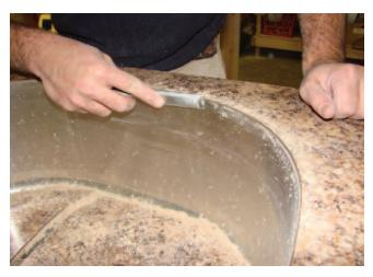
A chisel slid gently along the bowl wall just under the laminate helps to remove adhesive from the sink wall.
