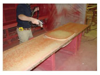
Lay the sink cutout over the sink and spray contact adhesive over the substrate.
