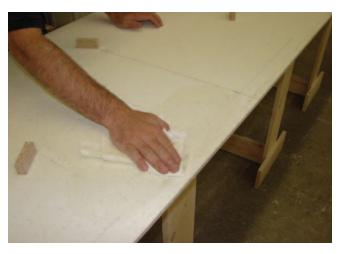
Clean the back of the solid surface where sink will adhere with a denatured alcohol. Remove all pencil lines.
