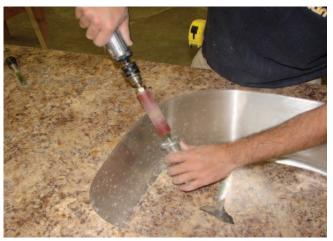
A 1" x 4" drum sander available from Karran along with an air drill is a good alternative to hand filing. Hold the drum sander at as much of a vertical angle as possible and run it backwards and forwards along the edge of the laminate. As soon as a slight glint of steel can be seen through the seam adhesive, stop sanding and remove remaining adhesive with a chisel as shown below.
