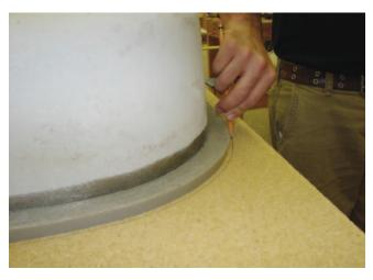
Place the sink upside down on the substrate in the marked position, then use a pencil to trace the outline of the sink onto the substrate. Hold your pencil vertically as this will offset your cutout line by the required 1/8".
