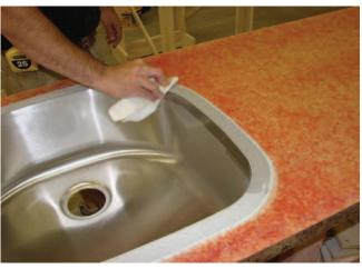
Clean the rim of the sink with denatured alcohol and a clean rag. Also clean the back of the laminate where the sink will attach with denatured alcohol.
