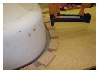
Flip the countertop over. Place sink in cutout to check for fit. Approximately 1/8" gap should be visible. Either screw or glue & staple wood support strips to the underside of the opening.
