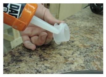
After drilling 1-1/2" holes for faucets, place a bead of silicone around wall of FHSR and slide into faucet hole. This will ensure your particleboard is completely sealed from possible water penetration.
