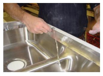
Place a strip of tape around the rim of the sink. Place strip 1/4" above rim then remove excess with a sharp blade. Ensure that no tape remains above rim of sink.
