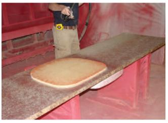
Place your sink cutout over the marked area on the back of laminate. This is done to protect this area of the laminate where the sink rim will bond from contact adhesive.
