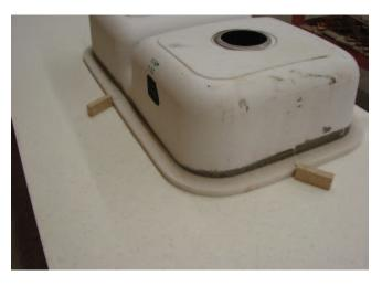
Place the sink upside down on the back of the solid surface in the marked position. Use hot melt glue to adhere blocks of wood to locate sink easily. Placing the corner of the block in line with the sink registration marks is simple and effective.
