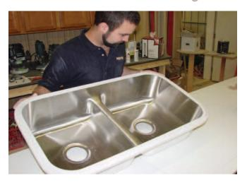
After removing the sink from its box, inspect it for damage.
