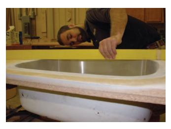
Check for level (low or high spots) after sanding is complete.
