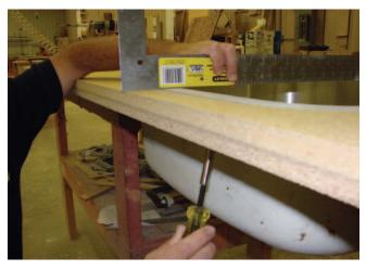
Flip the countertop and sink over. The sink rim must sit minimally higher than the top of the substrate. We recommend no more than 1/32". Adjust height as needed using either strips of laminate or screws. Regarding screws, simply position several screws around circumference of sink, screwed through the wood support strips until they touch the underside of rim. Then adjust screws to raise or lower rim height. Remember to make sure the sink remains centered in the hole.
