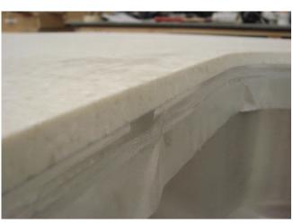
Final trimming should leave a slight overhang of solid surface and adhesive remaining.
