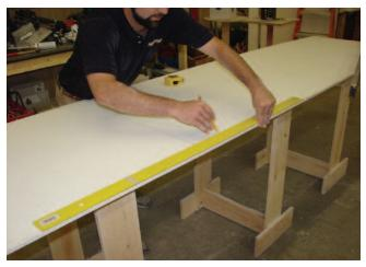
Measure and mark the back side of the solid surface countertop indicating where the sink needs to be installed. A set back from the front edge of 2" to 2-1/2" is recommended but always take into consideration the specific circumstances of each installation relating to cabinet and plumbing placement.
