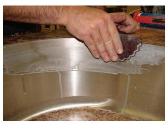
Polishing paste (available from Karran) along with a maroon Scotch-Brite pad will polish and finish sink wall if needed.
