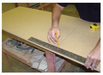
Measure and mark the back side of the countertop indicating where the sink needs to be installed. A set back from the front edge of 2" to 2-1/2" is recommended but always take into consideration the specific circumstances of each installation relating to cabinet and plumbing placement.
