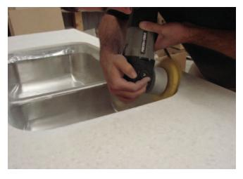
An orbital sander with a soft radius pad and 60 to 80 micron sandpaper should be used to sand the solid surface back to the bowl wall.
