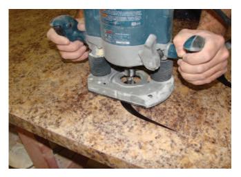
Use a router with an overhang bit or straight trim bit with oversized nylon bearing to remove laminate from the interior of the bowl. This is a commonly used bit to rough cut out acrylic sinks in solid surface.
